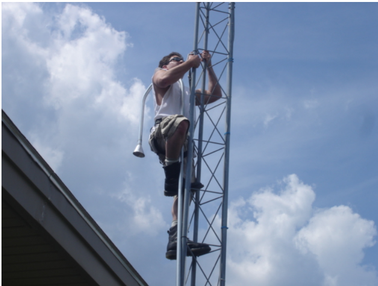
Installing a new ozone inlet.
