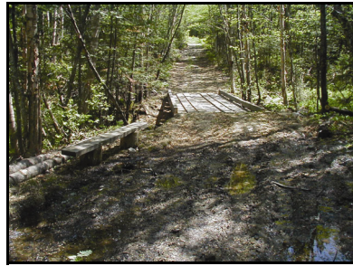
AFTER: An improved bridge prevents soil from entering the stream and reduces habitat destruction.
