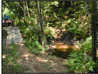
BEFORE: An inadequate bridge over the stream encouraged ATVs to go through it instead.
