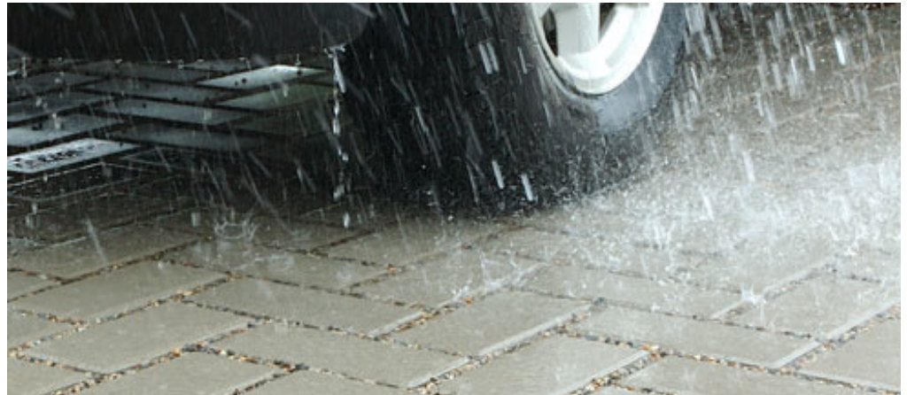
Illustrating the ability of rain to flow into the spaces between the pavers and not remain on top.
